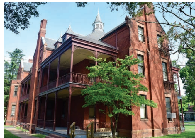
Slated for renovation, Westminster Hall is the third of the three original campus buildings on the Richmond campus. It features an array of exterior porches and cast-iron balconies.
