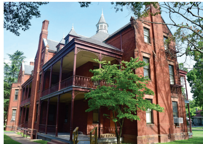
Slated for renovation, Westminster Hall is the third of the three original campus buildings on the Richmond campus. It features an array of exterior porches and cast-iron balconies.
